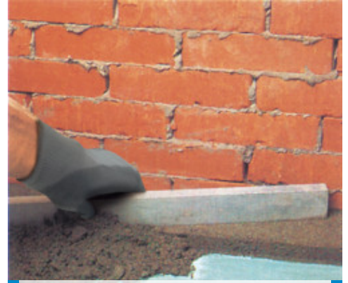
Application of cementitious screed with Planicrete admix
