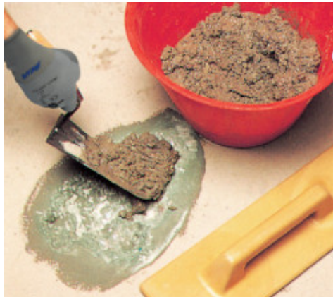
Floor patching: application of mortar
