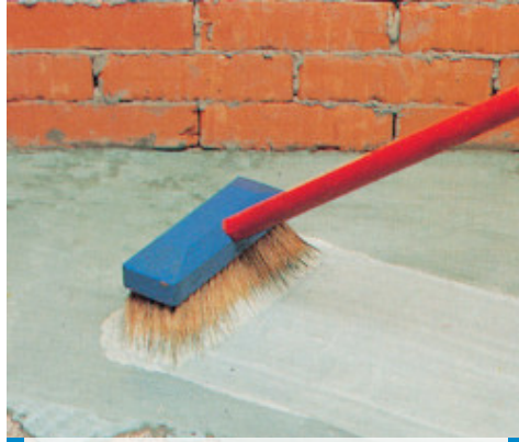
Application of cementitious grout with Planicrete admix
