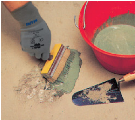
Floor patching: application of slurry
